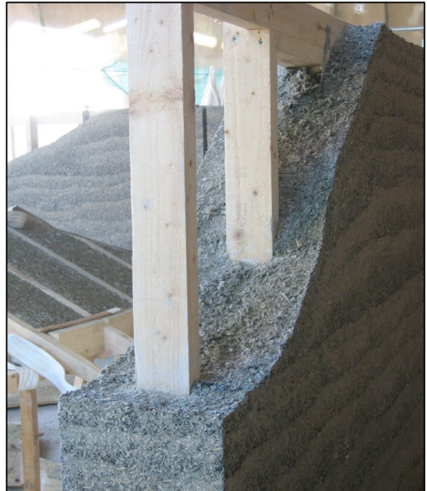
Figure 2.7 - Lime-hemp on a timber frame
